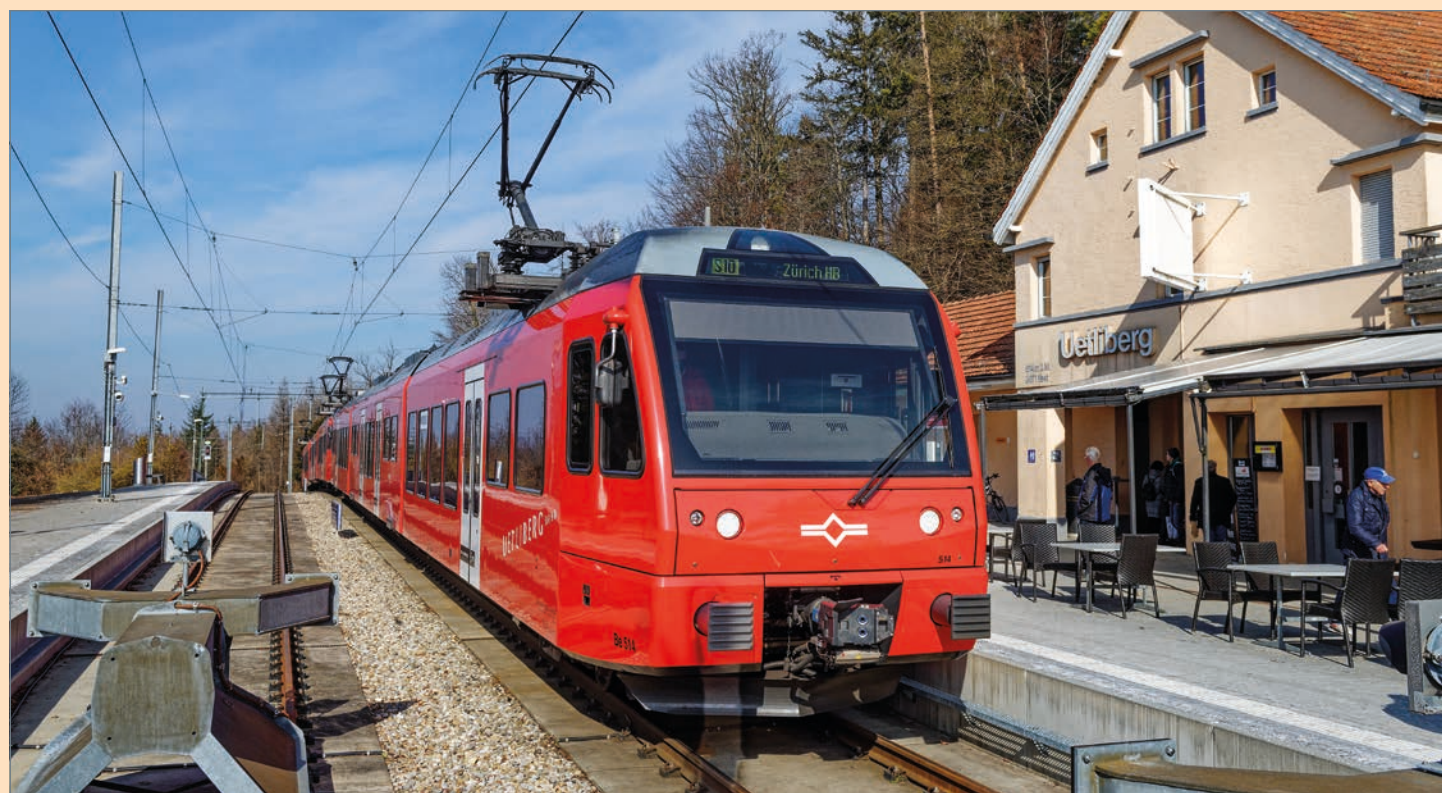
After the conversion of the Uetlibergbahn line to AC operation has been completed, only Class Be 552 multiple units will run up the Uetliberg. These trains are already equipped for both power systems, for the old DC- and the new AC-system. Six such trains (Be 552 511–516) were delivered in 2013/2014 and five more (Be 552 571–575) are currently in course of delivery. All the older trains are being withdrawn. Be 522 514 is seen at Uetliberg station on 8 March 2022.
