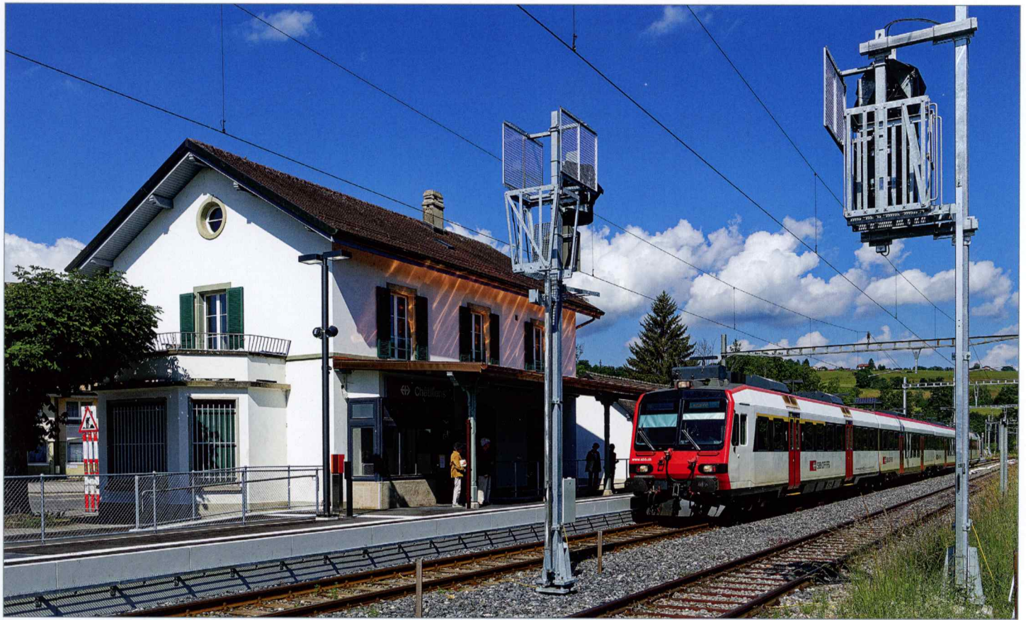
The completely remodelled Châtillens station has a raised platform and a newly built crossing track, which is only used by passing goods trains. 13 June 2024.
