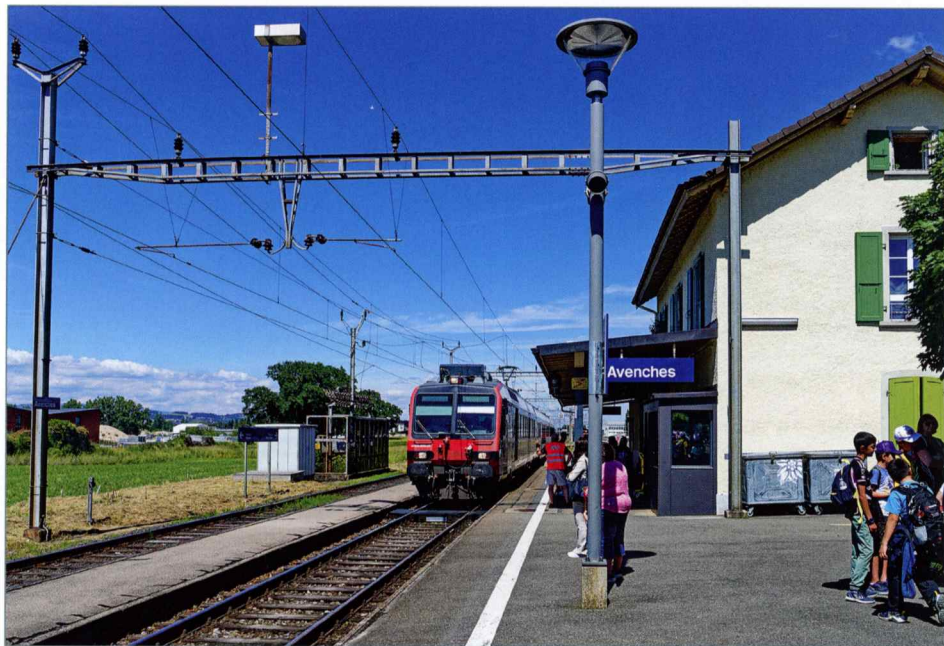
On 13 June 2024, a Domino train arrives at Avenches station, the loop of which has not yet been extended. As soon as the train stops, the crossing train enters the loop. Boarding and alighting is not entirely safe for passengers, especially for disabled people, as the platforms are not yet raised. In Roman times, the most important city on Swiss soil was located here, in what was then Aventicum! With its Roman ruins, the Musée Romain, which is well worth a visit, and the historic old town, Avenches has a number of sights to offer.
